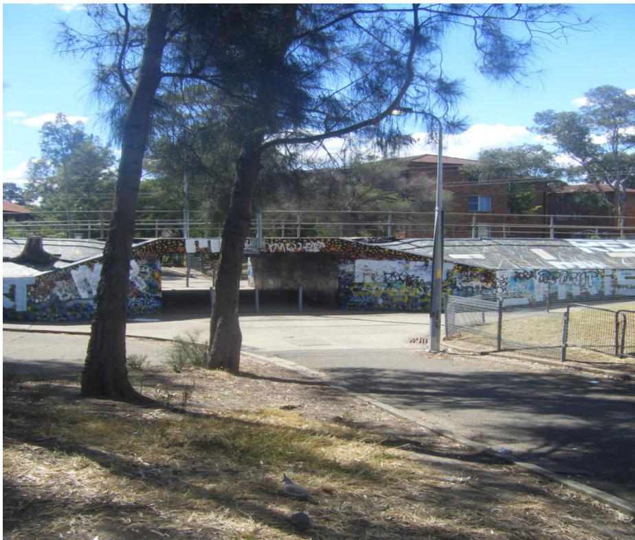
Figure 11: Traffic Bridge and Tunnel
