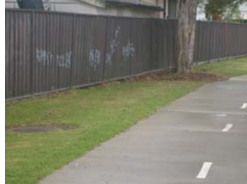
5.107 Graffiti on fence boundary
