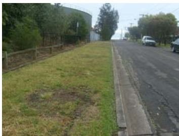
5.77: Wide but uneven footpath
