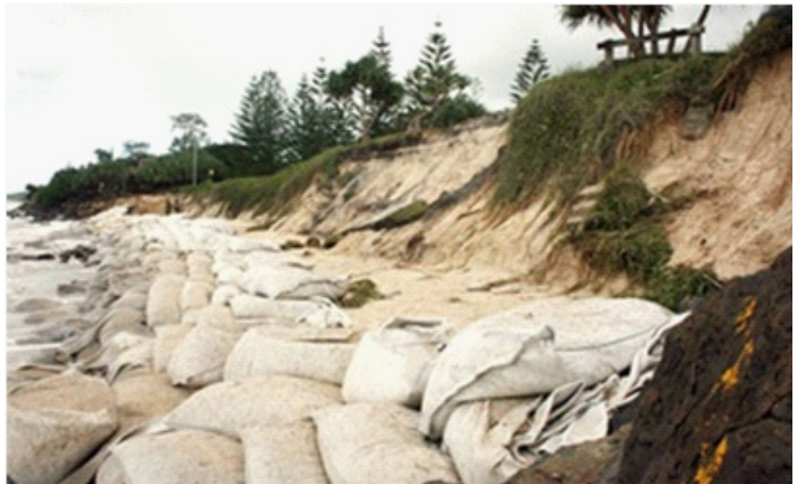
Figure 16: Illegal sandbagging along Belongil Beach, Byron Bay. (Source: Byron Shire News 2009)
