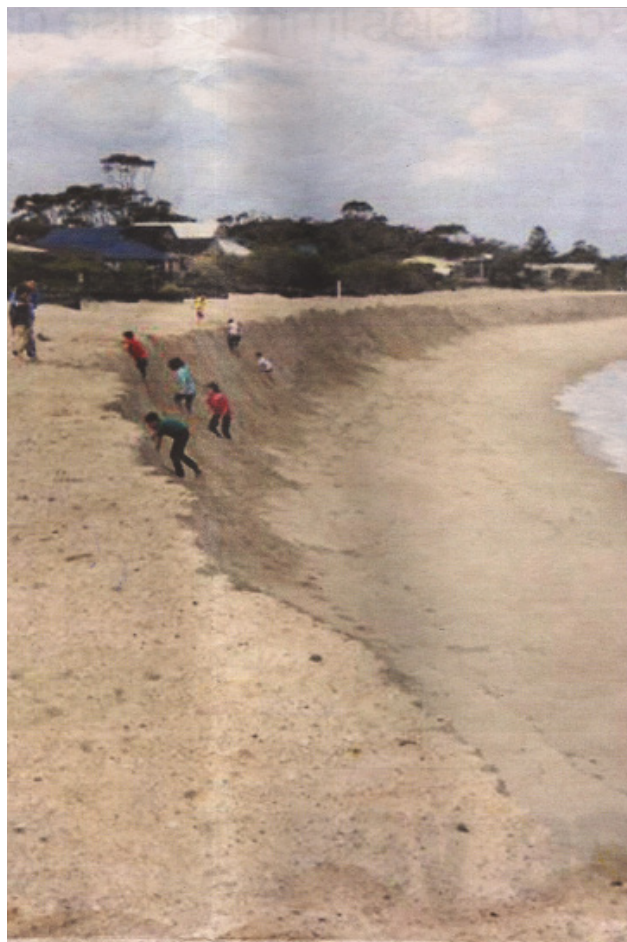
Figure 12: One day of massive seas has undone $307,000 of sand replenishment at Jimmy's Beach on the mid north coast of NSW. (Source: Campbell 2009).
