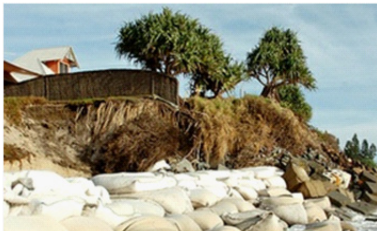
Figure 15: Residents along Belongil Beach, Byron bay, have dumped sandbags on the seaward side of their properties to stop them being washed into the sea. (Source: Tondorf 2009)
